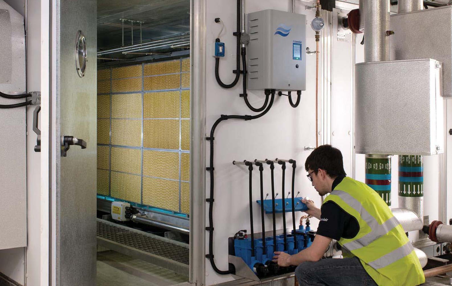
Condair ME with externally mounted hydraulic unit
