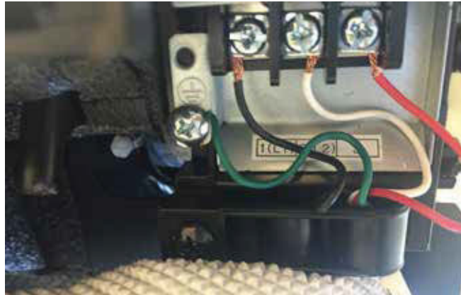
Figure 6-8 Indoor-unit terminal block with grounding cable (example only)
