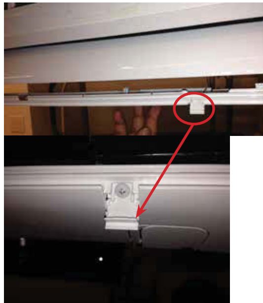
Figure 6-4 Latch over the screws on bottom panel of indoor unit
