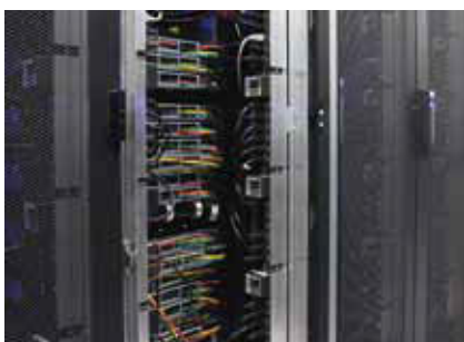
Knürr® DCM server rack for cooling with Liebert® DCL, Liebert® power distribution modules and integrated cable management.
